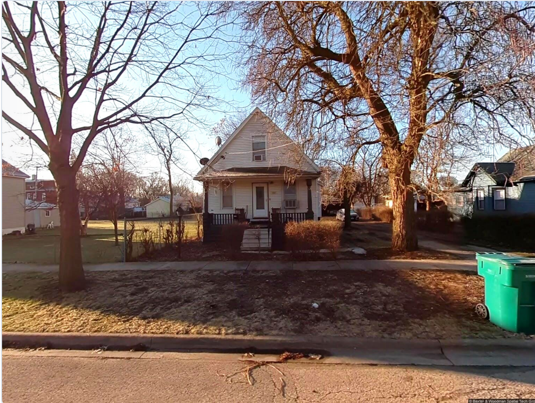
The house from Chase Avenue. Covered front porch, detached garage at the rear.
